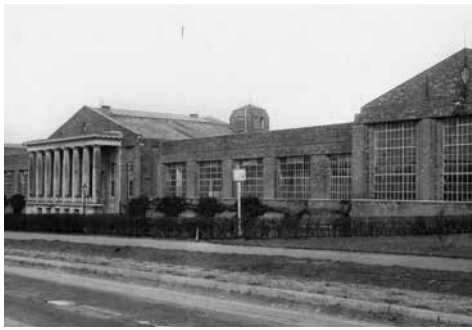
Rheinische Metallwaren- und Maschinenfabrik in Düsseldorf where the Kaiser-Wilhelm-Institut für Eisenforschung was located from 1920 until 1935.
